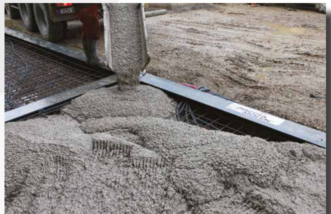
Concrete pouring that can be carried out by yourself.
